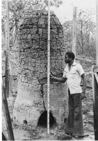
Figure 0.4. The down-draught iron smelting furnace near Kasungu, Malawi. The stack is made of baked clay taken from termite mounds and is sufficiently high to permit the furnace to attain smelting temperature by natural draft rather than with an air blast provided by pumping bellows. Source: David J. Killick, used with permission.
