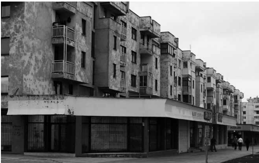
FIGURE 0.2. A Dobrinja building several years after reconstruction (photo by Vanja Čelebičić, 2010)
