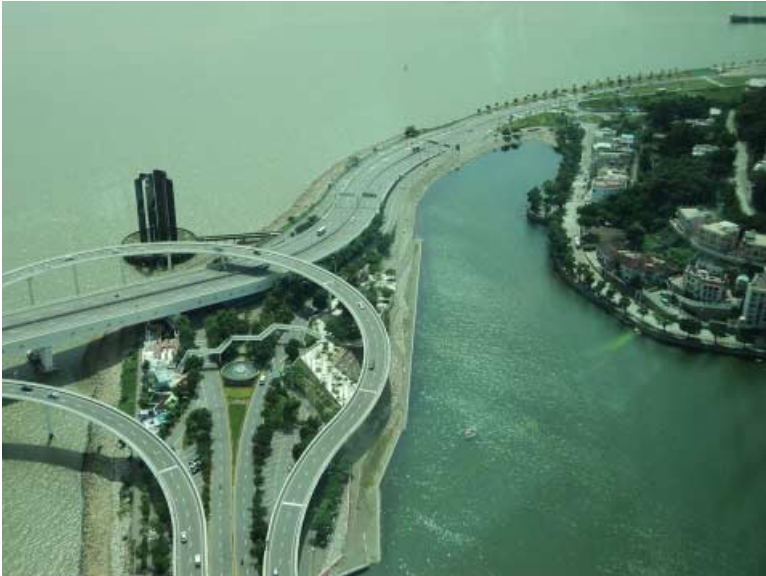
Figure 0.2. Panoramic view of Republic Avenue and the Sai Van lake, Macao 2010. The image shows one end of the eponymous third and final bridge linking Macao and Taipa. Concluded in 2004, it is the only suspension bridge in Macao and has two levels, an upper and a lower level, which operate even during bad weather and has set up the infrastructure to accommodate Macao’s light rail metro system currently operating just in Taipa. Photo by the author.
