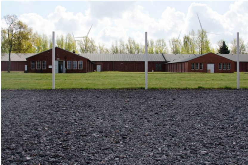
Figure 4.7. View of the building of the former Walther-Werke at the Neuengamme Memorial © Emily Mohney/Neuengamme Memorial
