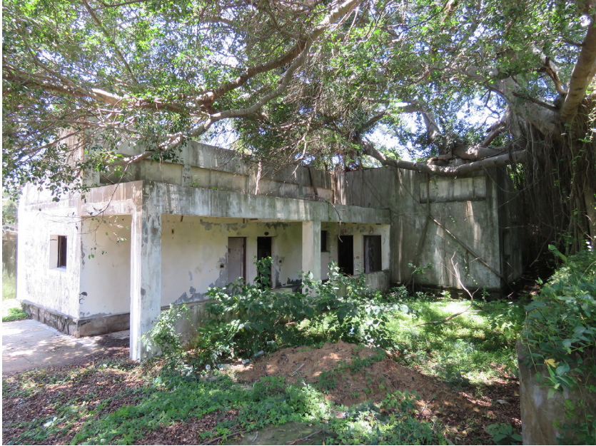
Figure 2.1. A disused building of a former military brothel in Anqian, Kinmen, 2018. © Hsiao-Chiao Chiu.
